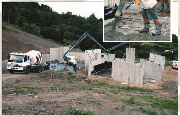
Work in progress: Retaining fence nearing completion. Tilt slabs in place and concrete floor being poured.
