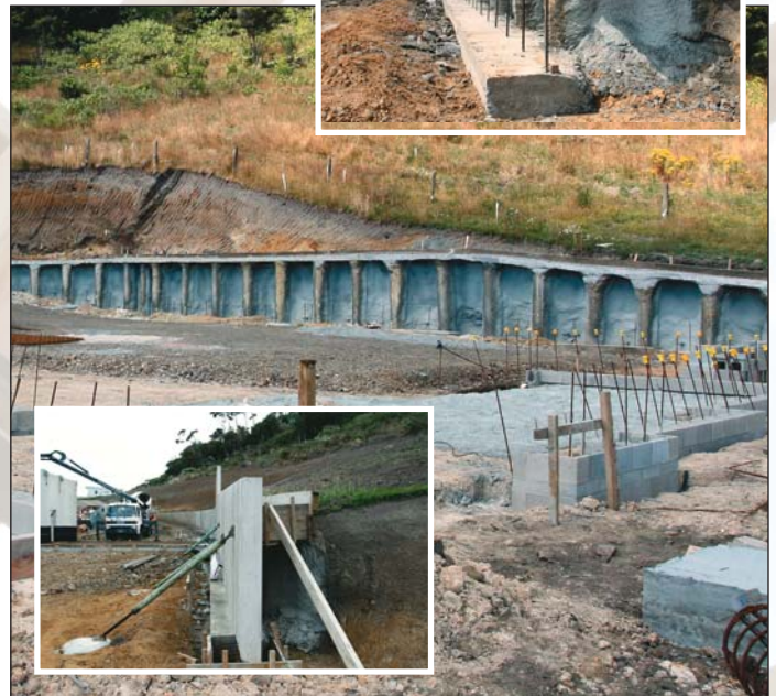
Work in progress: Retaining fence nearing completion. Tilt slabs in place and concrete floor being poured.
