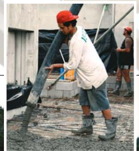
Work in progress: Retaining fence nearing completion. Tilt slabs in place and concrete floor being poured.
