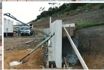
Work in progress: Retaining fence nearing completion. Tilt slabs in place and concrete floor being poured.
